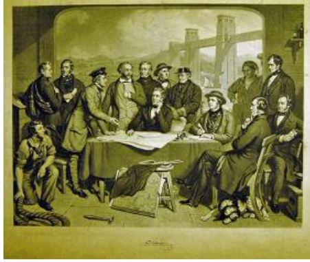
Engraving. Conference of Engineers at the Menai Straits preparatory to floating one of the tubes of the Britannia Bridge. Signed by Robert Stephenson. Painted by John Lucas. Engraved by James Scott. Published by Henry Graves & Company, Printsellers to the Queens, 6 Pall Mall, London. 25 January 1858.
